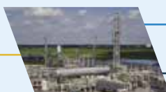
NATURAL GAS PROCESSING PLANT
