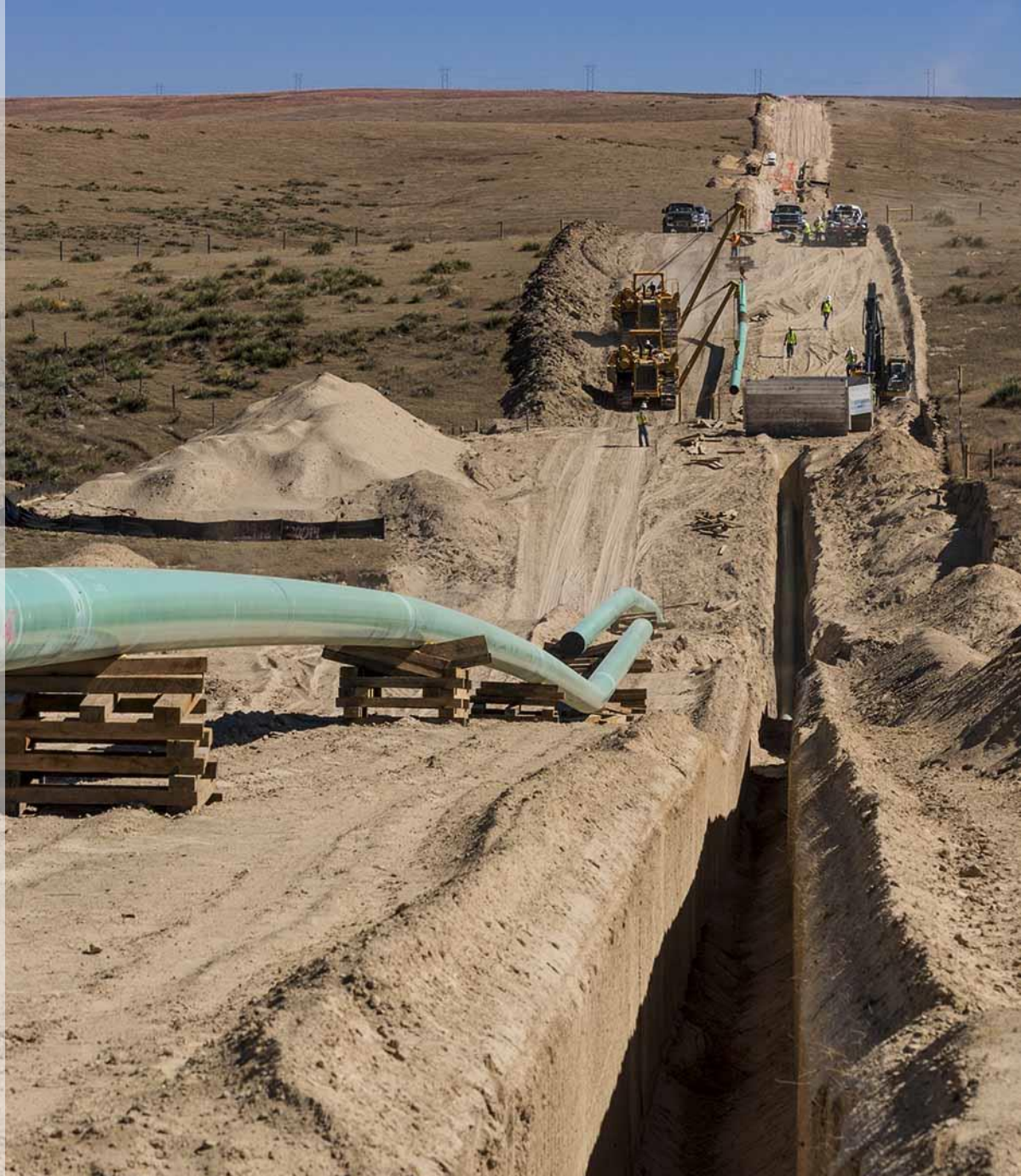
Elk Creek Pipeline – Kansas
