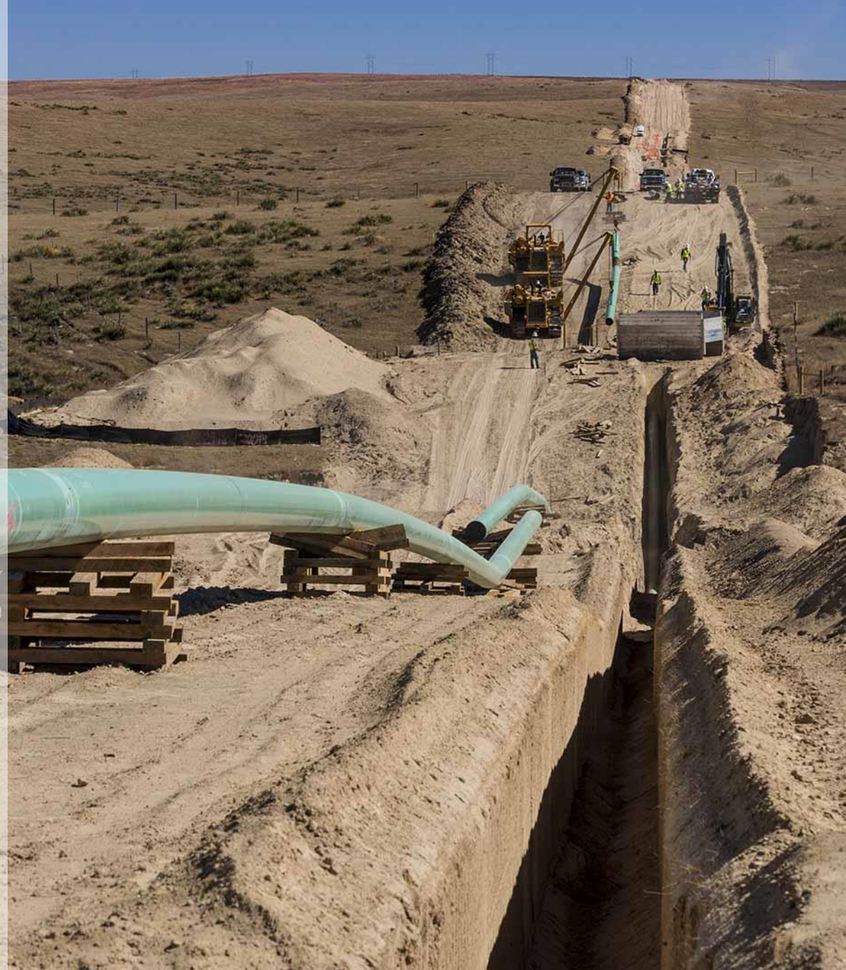
Elk Creek Pipeline – Kansas
