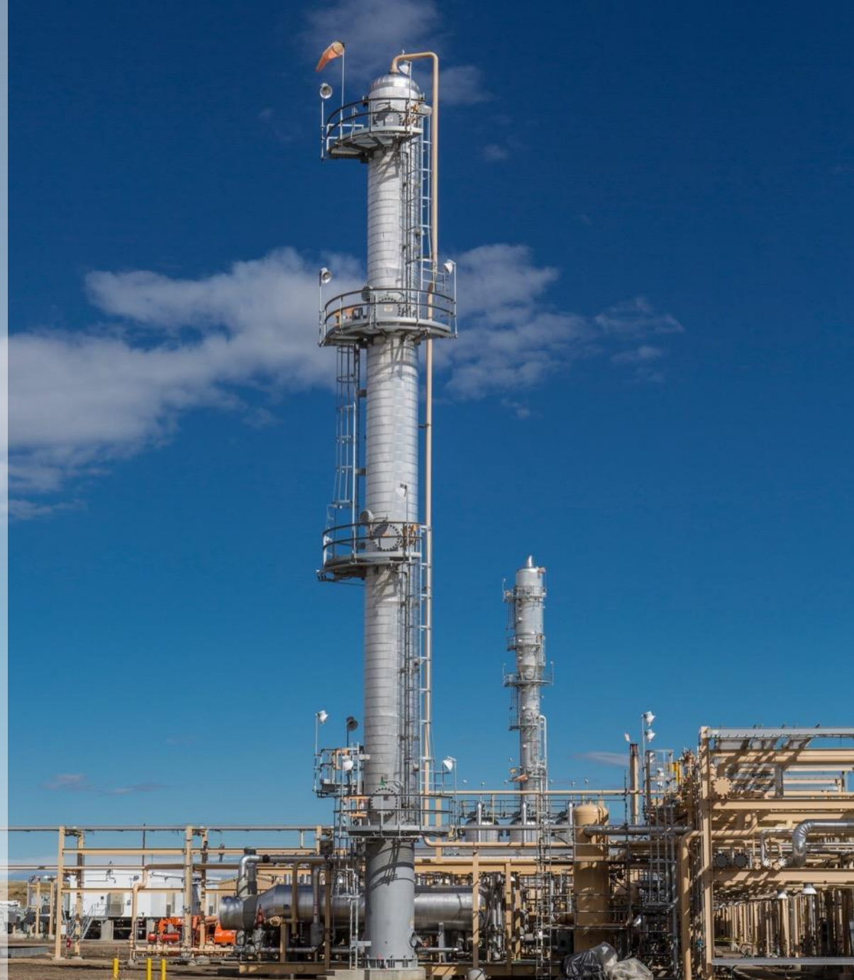
Bear Creek plant — Williston Basin
