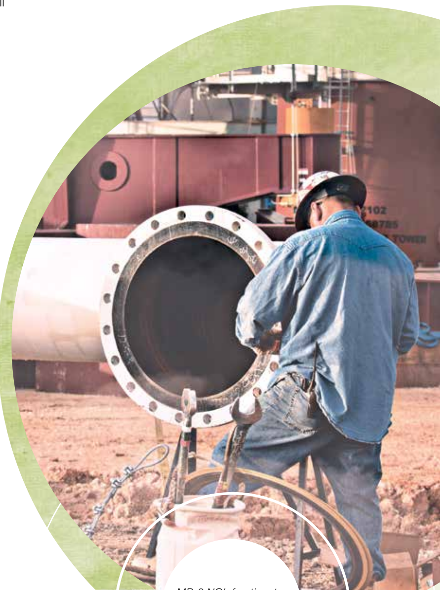
MB-3 NGL fractionator under construction in Mont Belvieu, Texas.
