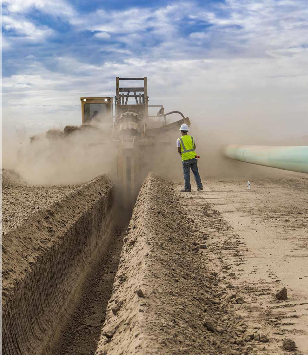
Elk Creek Pipeline – Wyoming
